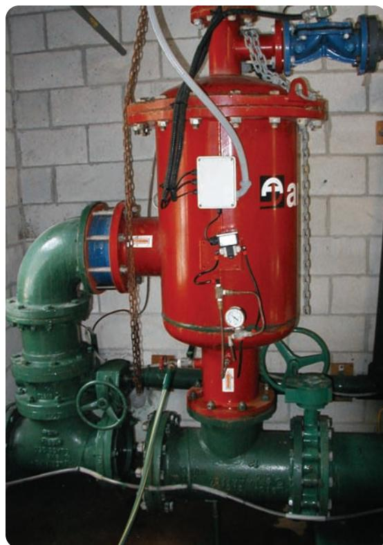
An automatic self-cleaning filter system such as this one at the point of entry can prevent problems due to sediment.
