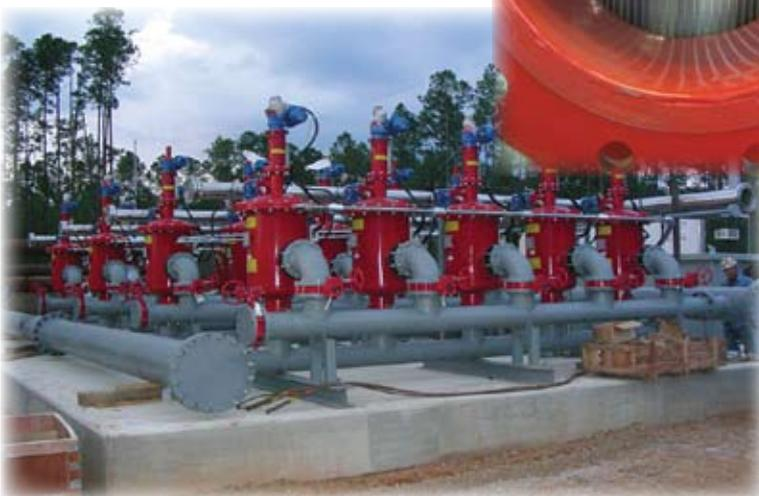
Filtering particulates from process water reduces plugging in the formation that is reached by deep disposal wells.
