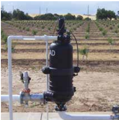
Canal water, 250 gpm, 200 micron, protecting jet sprinklers
