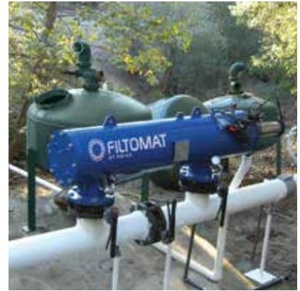
Reservoir water, 400 gpm, 100 micron, protecting drip irrigation
