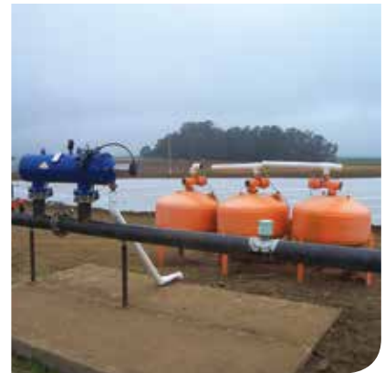
Well water, 500 gpm, 80 micron, protecting drip tape irrigation
