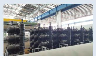
**Stage 1** Filters: 22 units of 4 x 10" Super Galaxy vertical modules Filtration degree: 100 micron Flow rate: 13,900 m<sup>3</sup>/h – 61,160 gpm
