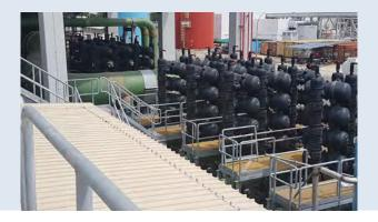
**Stage 2** Filters: 34 units of 4 x 10" Super Galaxy vertical modules Filtration degree: 20 micron Flow rate: 12,800 m<sup>3</sup>/h – 56,320 gpm
